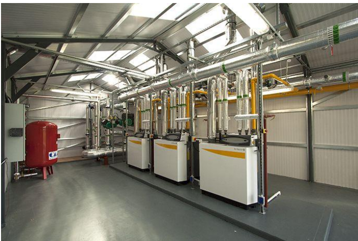
Primary Reverse Return Header System Incorporating Wilo Circulators.
