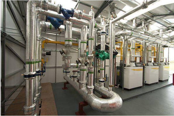
Primary Reverse Return Header System Incorporating Wilo Circulators.
